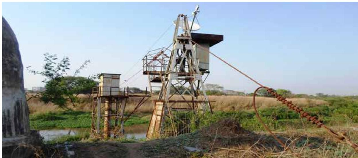
FIGURE 3.23 (B): A MANUALLY OPERATED CABLEWAY INSTALLED IN MAHARASHTRA
