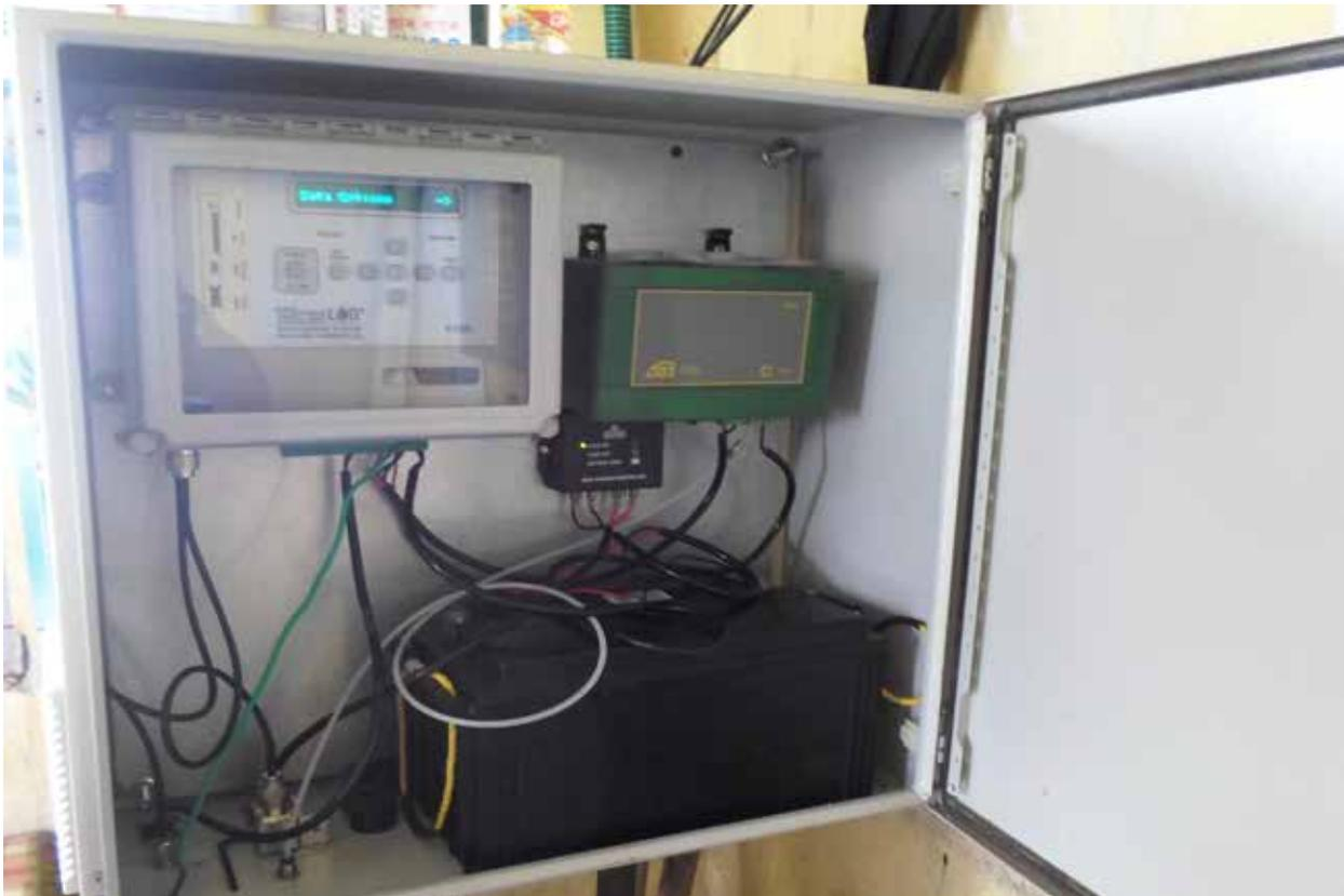
**FIGURE 3.12: A BUBBLER SYSTEM INSTALLED BY CWC IN GUWAHATI, ASSAM**
